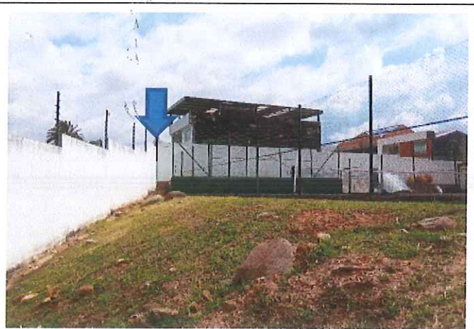
VISTA GENERAL AREA REQUERIDA
