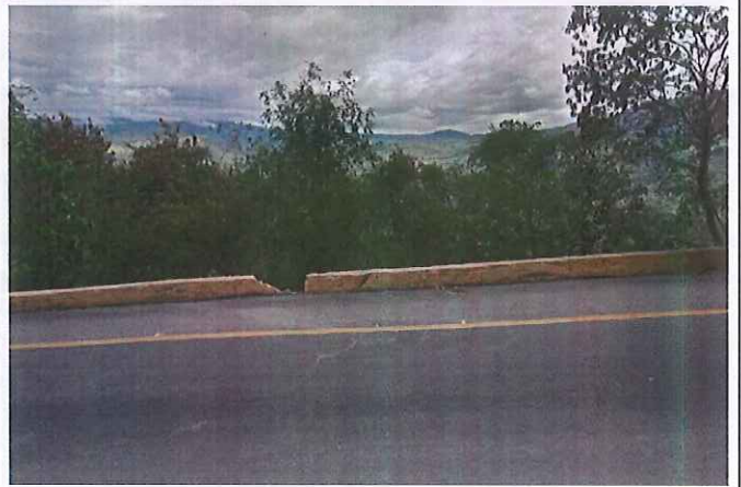
VISTA GENERAL AREA REQUERIDA 8
